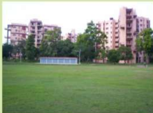
Residential Complex & Football Ground
