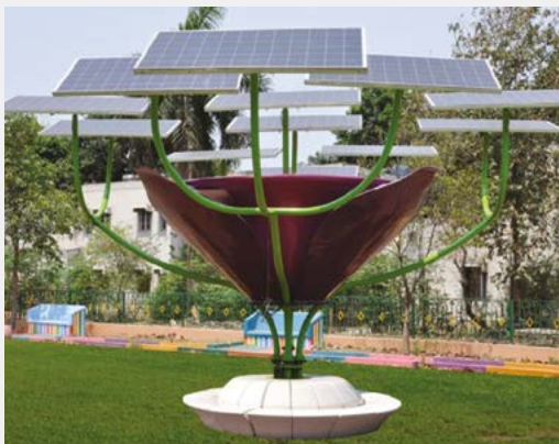
Figure 2: 3.6 kWp Solar Lotus installed at Children Park, CMERI Colony
