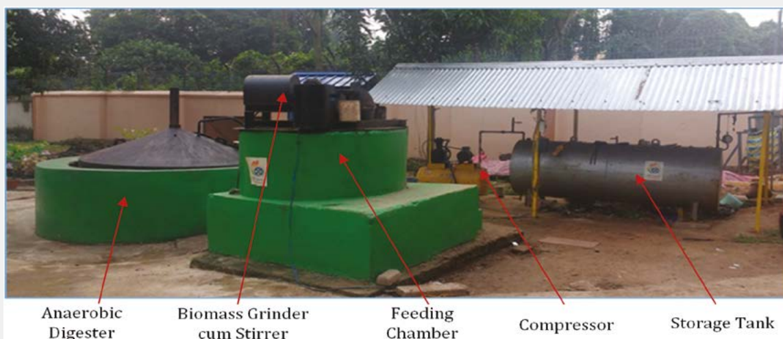
Figure 12: Bio-methanation Unit of 10 cum capacity at CSIR-CMERI
