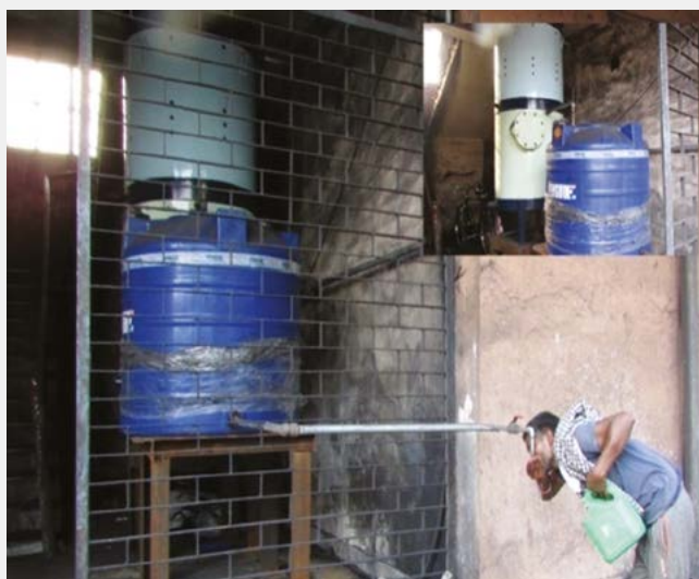
Iron removal plant installed at M/s Satyam Smelters Pvt. Ltd, Jamuria (attached with submersible pump)
