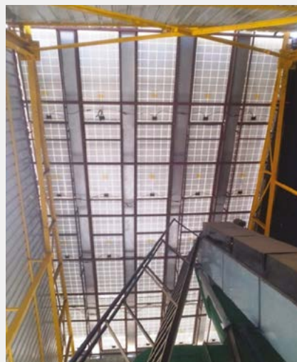
Figure 4: 7.5 kWp Solar Roof installed at MSW Complex, CMERI Colony
