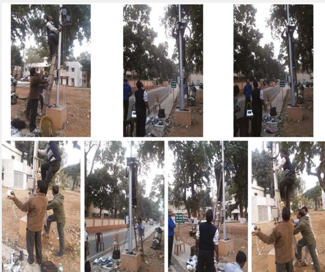
Figure 7: Setup for live vehicle detection on-site: Tasks include Installation of camera, enclosure with entire hardware with onboard software
