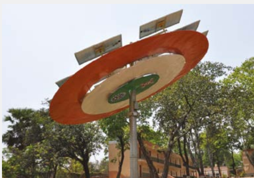
Figure 3: 5.4 kWp Solar Tree installed at the Guesthouse Complex, CMERI Colony
