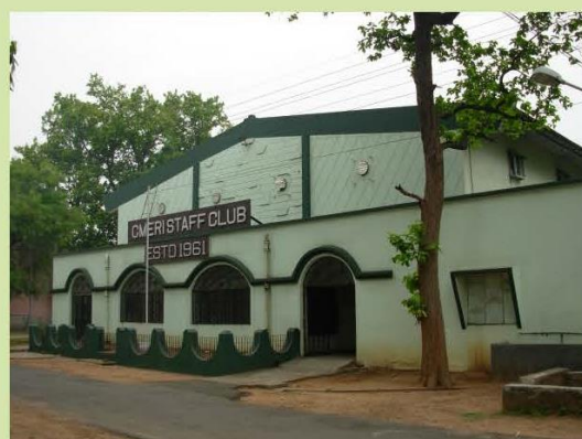
CMERI Staff Club Auditorium with indoor badminton courts
